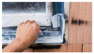
7. Install the AEROSANA FLEECE sub-sill flashing
