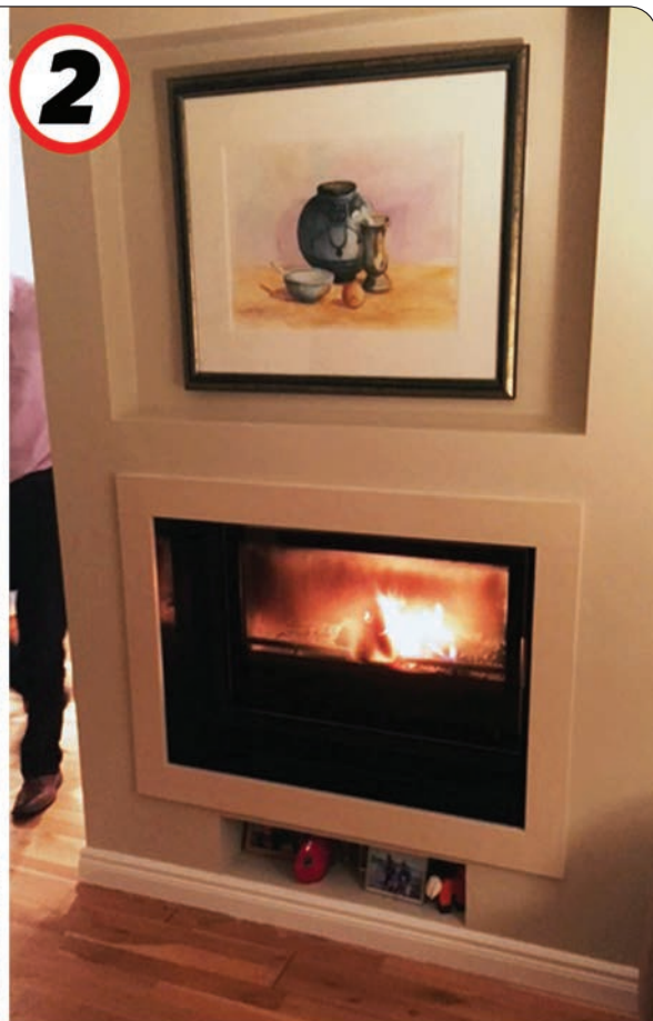
- COMPLETED INSTALL USING METAL STUD FRAME & HEAT RESISTANT PLASTERBOARD
